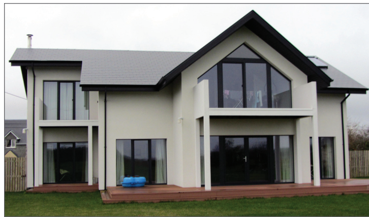
21.24 Shading devices: roof overhangs and balconies are both used in this house, built by Cyril Mannion in Athenry, Co. Galway.
