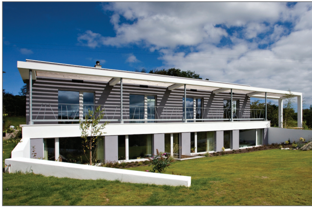
21.25 Shading devices: notice the striped shadow pattern cast by the brise soleil on the first floor façade on this house in Co. Wicklow.
