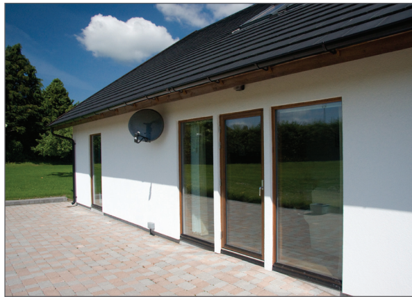
21.23 Shading devices: notice the shadow cast by the roof overhang on this home by Scandinavian Homes of Co. Galway.
